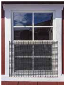
Wire Over Windows
